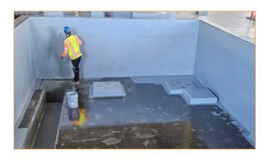
Protecto-Flex® high-build, glass-flake reinforced, epoxy and novolac epoxy coatings provide exceptional resistance to the harshest chemical exposures. Depending on their resin base and finished DFT, Protecto-Flex products are suitable for mild atmospheric exposure to exceptionally severe immersion service. Variants include products specially built for FDA compliance and high temperature exposure. It's what you specify when something more ordinary is not up to the task.
