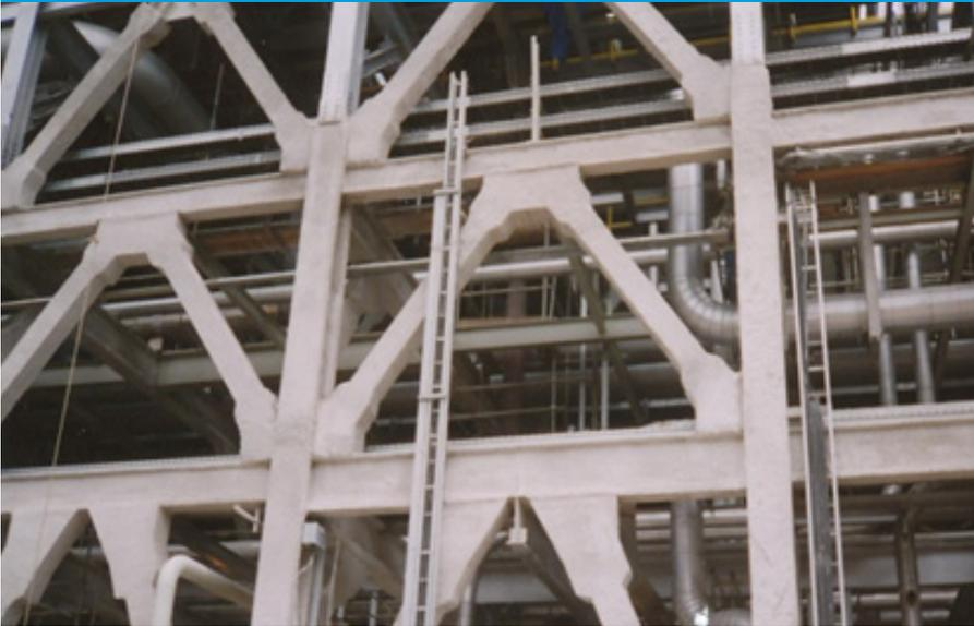
**Pyrocrete 40 is designed for the fire protection of exterior structural steel, vessel skirts, and for upgrading the fire resistance of any existing concrete. Pyrocrete 40 has highly competitive ratings for UL 1709, ASTM E119 and BS-476 (hydrocarbon curve) fire standards.**
