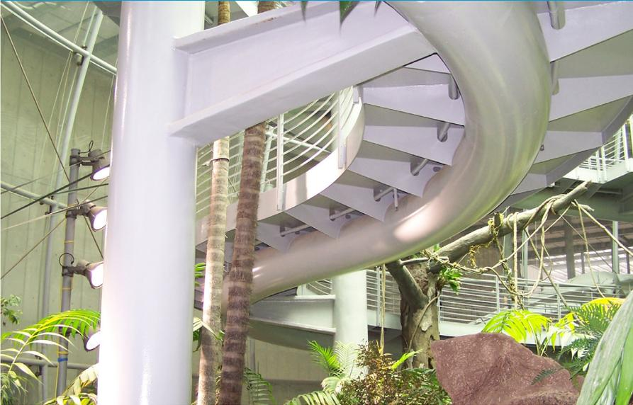
**A two component, architectural grade, epoxy based intumescent fireproofing coating which is spray applied directly to primed steel surfaces. Thermo-Lag 3000 is used to provide 1-3 hour cellulosic fire ratings for structural steel beams, columns, tubes, pipes, bulkheads and electrical raceways.**
