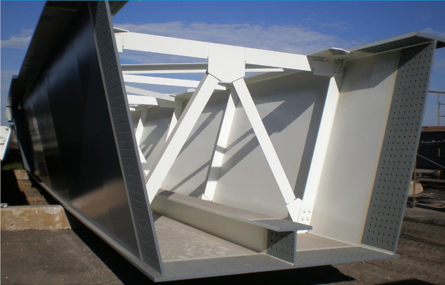
**Carbozinc 11 FC is a fast-cure inorganic zinc rich primer that allows topcoating in 4 hours at 75°F (24°C) and 60% relative humidity.**
