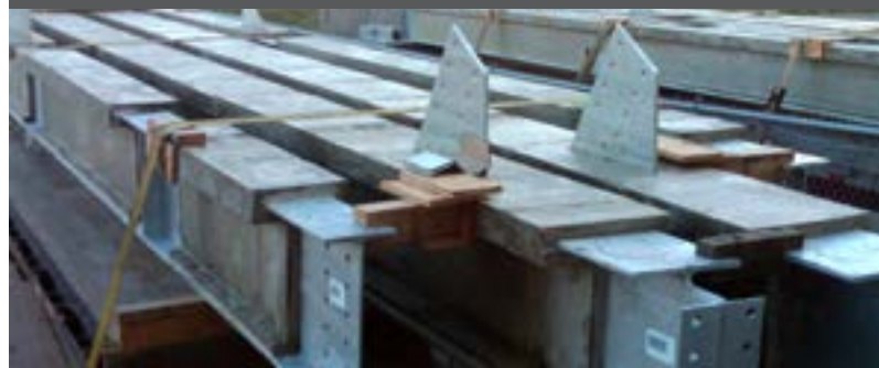
PYROCRETE 241 APPLIED OFFSITE AND TRANSPORTED TO JOBSITE.
